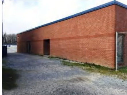
2). Northeast Elevation - Feb 08, 2017
