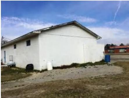
4). South Elevation - Feb 08, 2017
