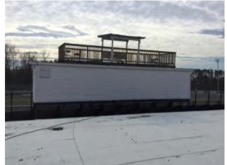
3). North Elevation - Feb 07, 2017
