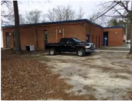
4). South Elevation - Feb 07, 2017
