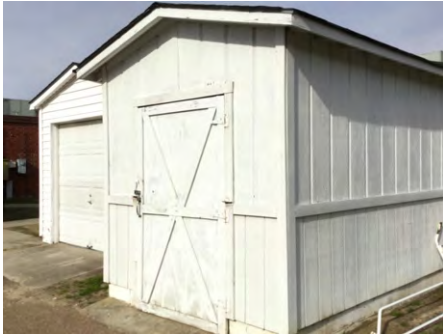
1). South Elevation - Feb 23, 2017
