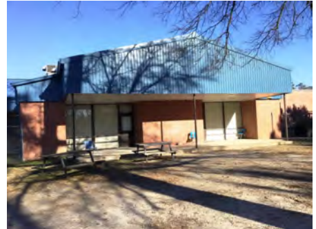
3). West Elevation - Feb 06, 2017
