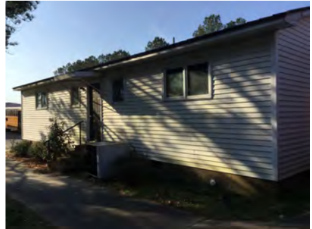
3). East Elevation - Feb 22, 2017
