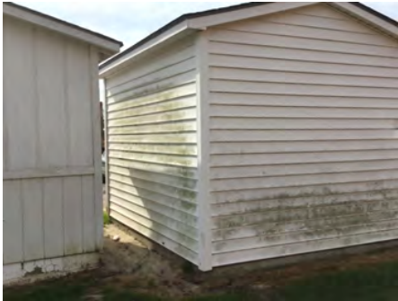
4). East Elevation - Feb 01, 2017
