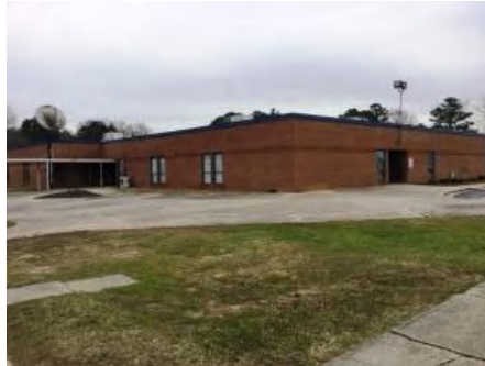
2). South Elevation - Feb 07, 2017
