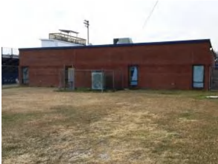
1). East Elevation - Feb 08, 2017
