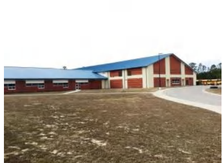
3). East Elevation - Feb 08, 2017
