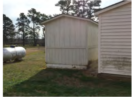
3). North Elevation - Feb 23, 2017
