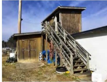
2). South Elevation - Feb 08, 2017
