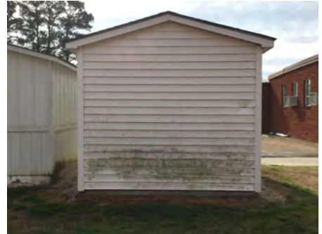
3). North Elevation - Feb 01, 2017
