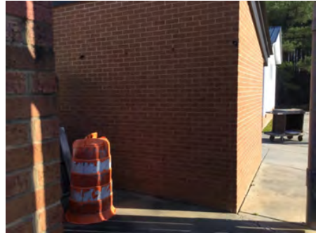
3). West Elevation - Feb 22, 2017
