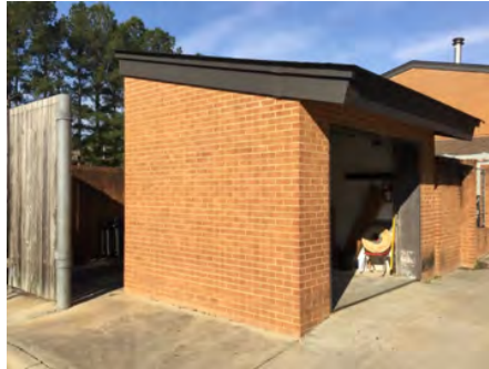
2). South Elevation - Feb 22, 2017
