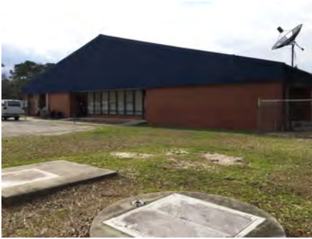
4). East Elevation - Feb 06, 2017
