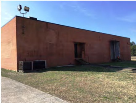
4). North Elevation - Feb 07, 2017
