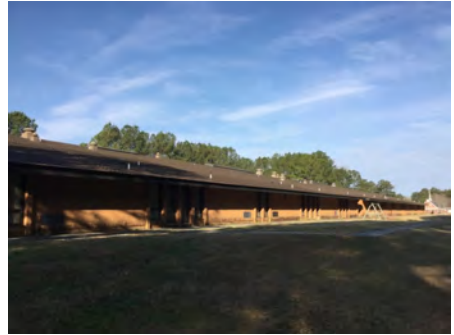
3). East Elevation - Feb 16, 2017
