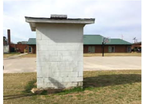
3). East Elevation - Feb 01, 2017
