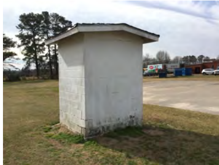
2). West Elevation - Feb 01, 2017
