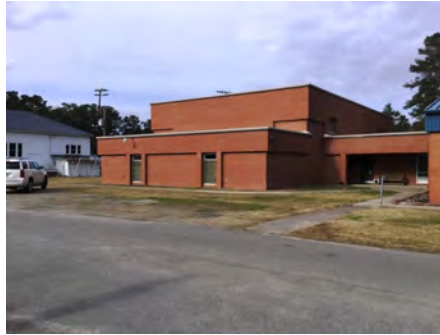
2). South Elevation - Feb 06, 2017
