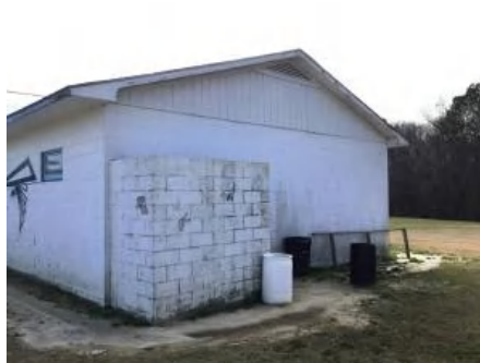
2). North Elevation - Feb 08, 2017
