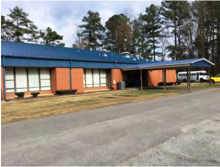
1). Southwest Elevation - Feb 06, 2017
