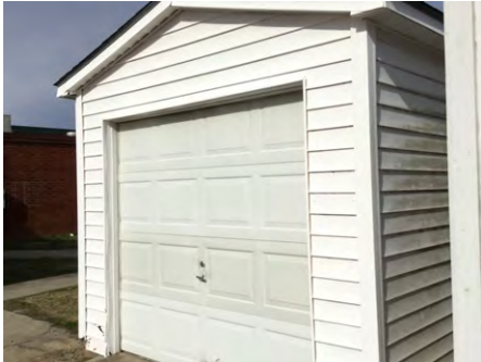
1). South Elevation - Feb 01, 2017
