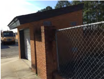
4). North Elevation - Feb 22, 2017
