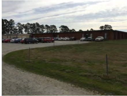
2). North Elevation - Feb 23, 2017
