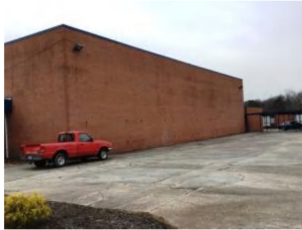
2). North Elevation - Feb 08, 2017
