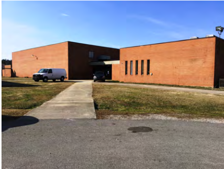
1). East Elevation - Feb 07, 2017
