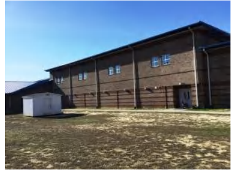
3). Northeast Elevation - Feb 08, 2017
