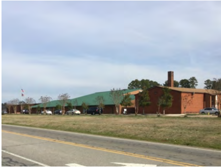
1). West Elevation - Feb 23, 2017
