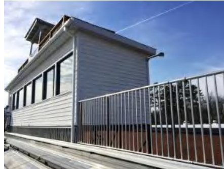
2). East Elevation - Feb 07, 2017
