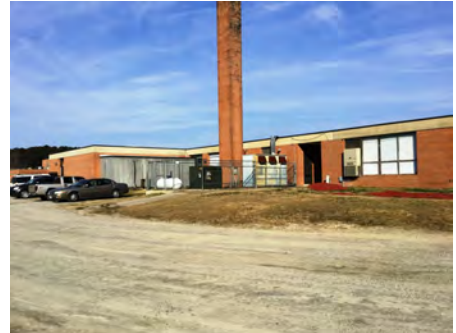
3). South Elevation - Feb 07, 2017
