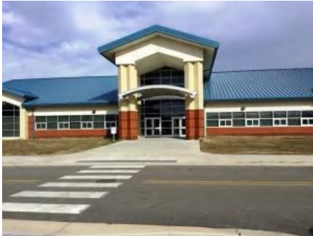
1). West Elevation - Feb 08, 2017
