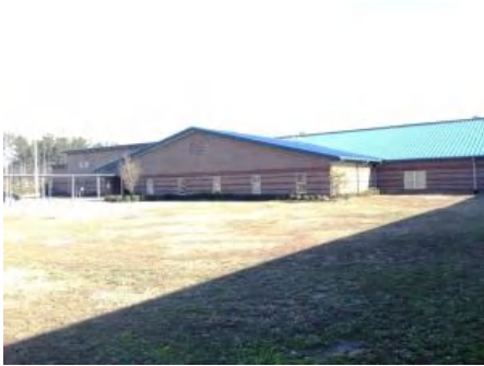
1). South Elevation - Feb 08, 2017
