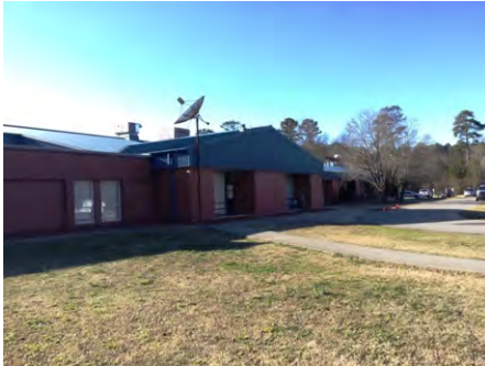
1). East Elevation - Feb 06, 2017
