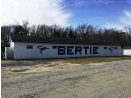
1). East Elevation - Feb 08, 2017
