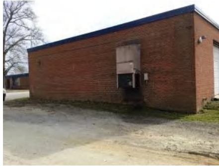
2). Northwest Elevation - Feb 07, 2017
