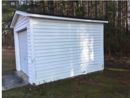
2). South Elevation - Feb 22, 2017
