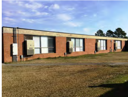
2). Northwest Elevation - Feb 07, 2017
