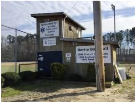
4). North Elevation - Feb 08, 2017
