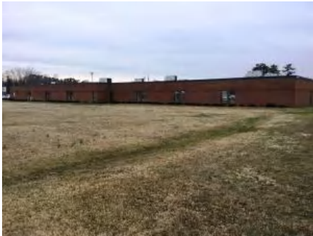
4). East Elevation - Feb 07, 2017
