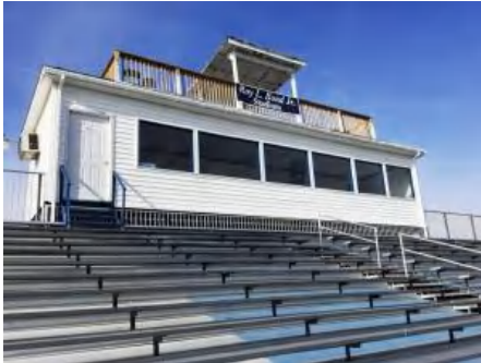
1). Southeast Elevation - Feb 07, 2017
