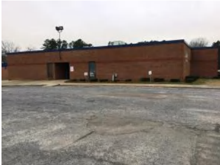
1). Southeast Elevation - Feb 07, 2017
