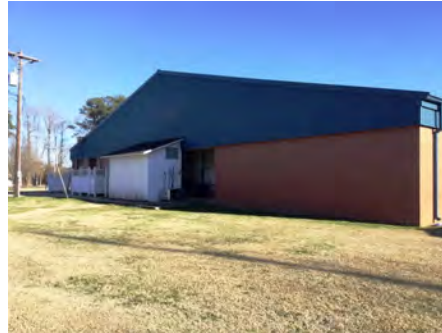
2). North Elevation - Feb 06, 2017
