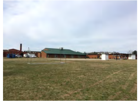
3). East Elevation - Feb 23, 2017
