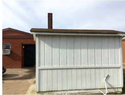
2). East Elevation - Feb 23, 2017
