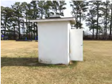
4). North Elevation - Feb 01, 2017
