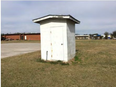
1). South Elevation - Feb 01, 2017
