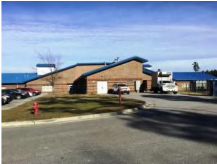
4). East Elevation - Feb 08, 2017
