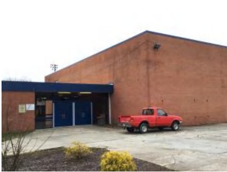
1). Northeast Elevation - Feb 08, 2017
