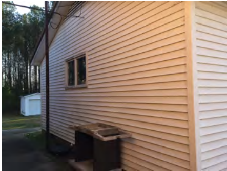
4). North Elevation - Feb 22, 2017
