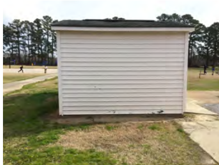
2). West Elevation - Feb 01, 2017
