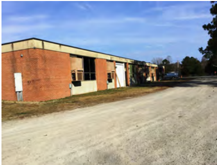
4). East Elevation - Feb 07, 2017
