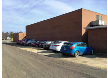
3). West Elevation - Feb 07, 2017
