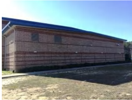
2). North Elevation - Feb 08, 2017
