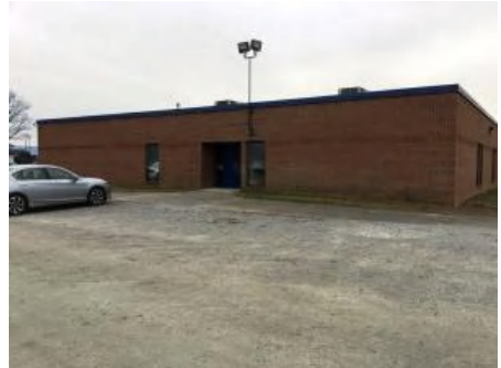
3). Northwest Elevation - Feb 07, 2017
