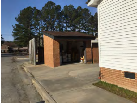
1). East Elevation - Feb 22, 2017
