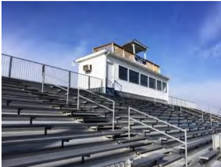
4). Southwest Elevation - Feb 07, 2017
