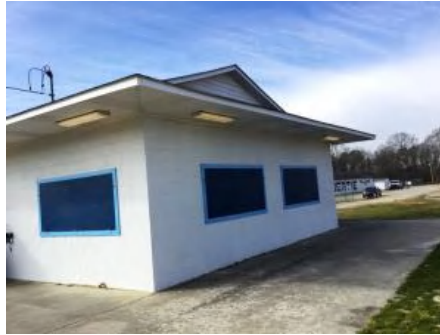
2). Southeast Elevation - Feb 08, 2017
