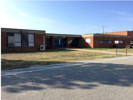
1). North Elevation - Feb 07, 2017
