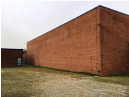
4). Southeast Elevation - Feb 08, 2017
