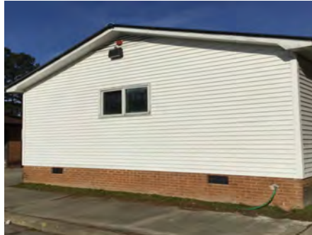
2). South Elevation - Feb 22, 2017
