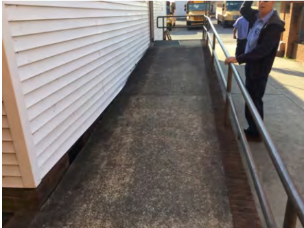
1). West Elevation - Feb 22, 2017
