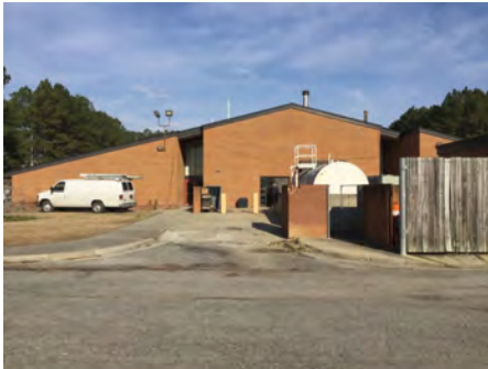
4). South Elevation - Feb 16, 2017
