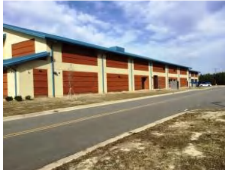
2). South Elevation - Feb 08, 2017
