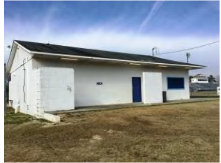
3). South Elevation - Feb 08, 2017
