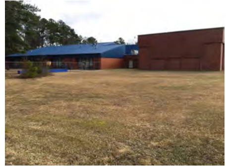
3). North Elevation - Feb 06, 2017
