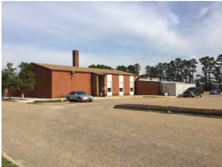
4). South Elevation - Feb 23, 2017
