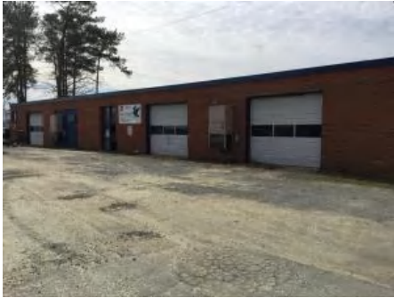
1). North Elevation - Feb 07, 2017
