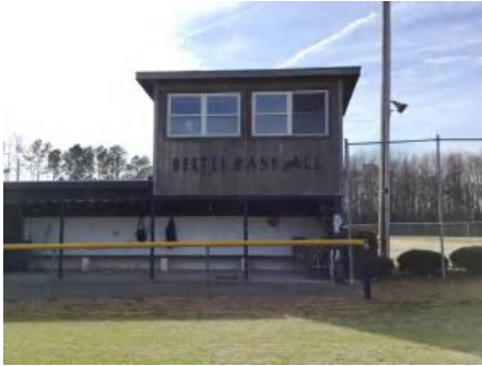
1). East Elevation - Feb 08, 2017
