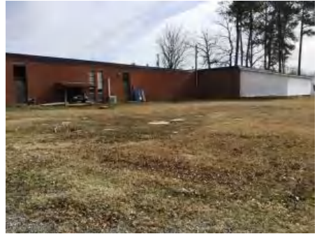
3). West Elevation - Feb 07, 2017
