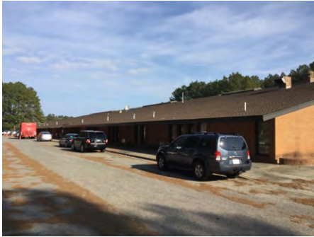
1). West Elevation - Feb 16, 2017
