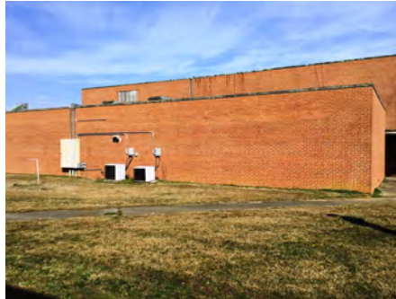
2). South Elevation - Feb 07, 2017
