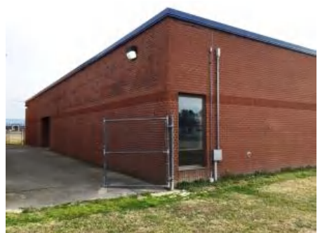
3). Northwest Elevation - Feb 08, 2017
