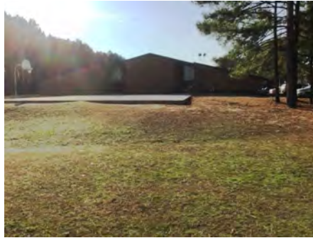
2). North Elevation - Feb 16, 2017
