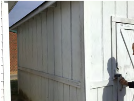
4). West Elevation - Feb 23, 2017
