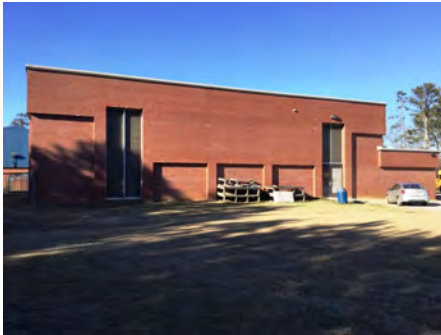
4). South Elevation - Feb 06, 2017
